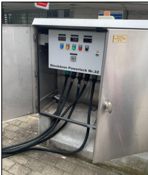
Figure 1: OPS facility for river cruise ships. Photograph by project team members, 2024. Basel, Switzerland.
