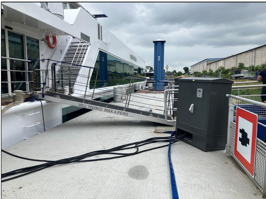
Figure 2: Shore-side eco-power for river cruise ships in Bamberg. Photograph, 2023. Bayernhafen, Bamberg, Germany.
