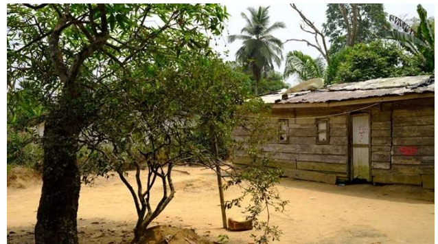
Figure 3: Typical house in Pitti
