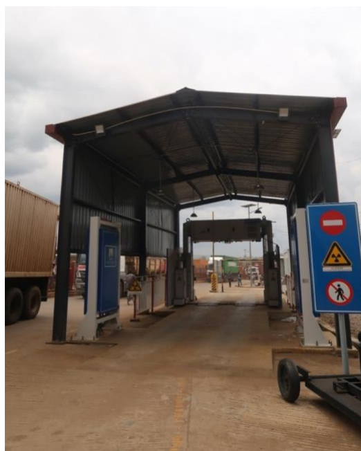
Figure 10: Scanning system at the Malaba OSBP
