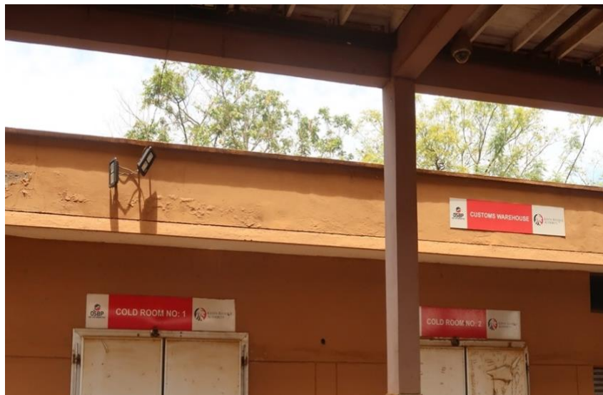
Figure 12: Cold storage infrastructure at the Malaba OSBP (Kenyan side)
