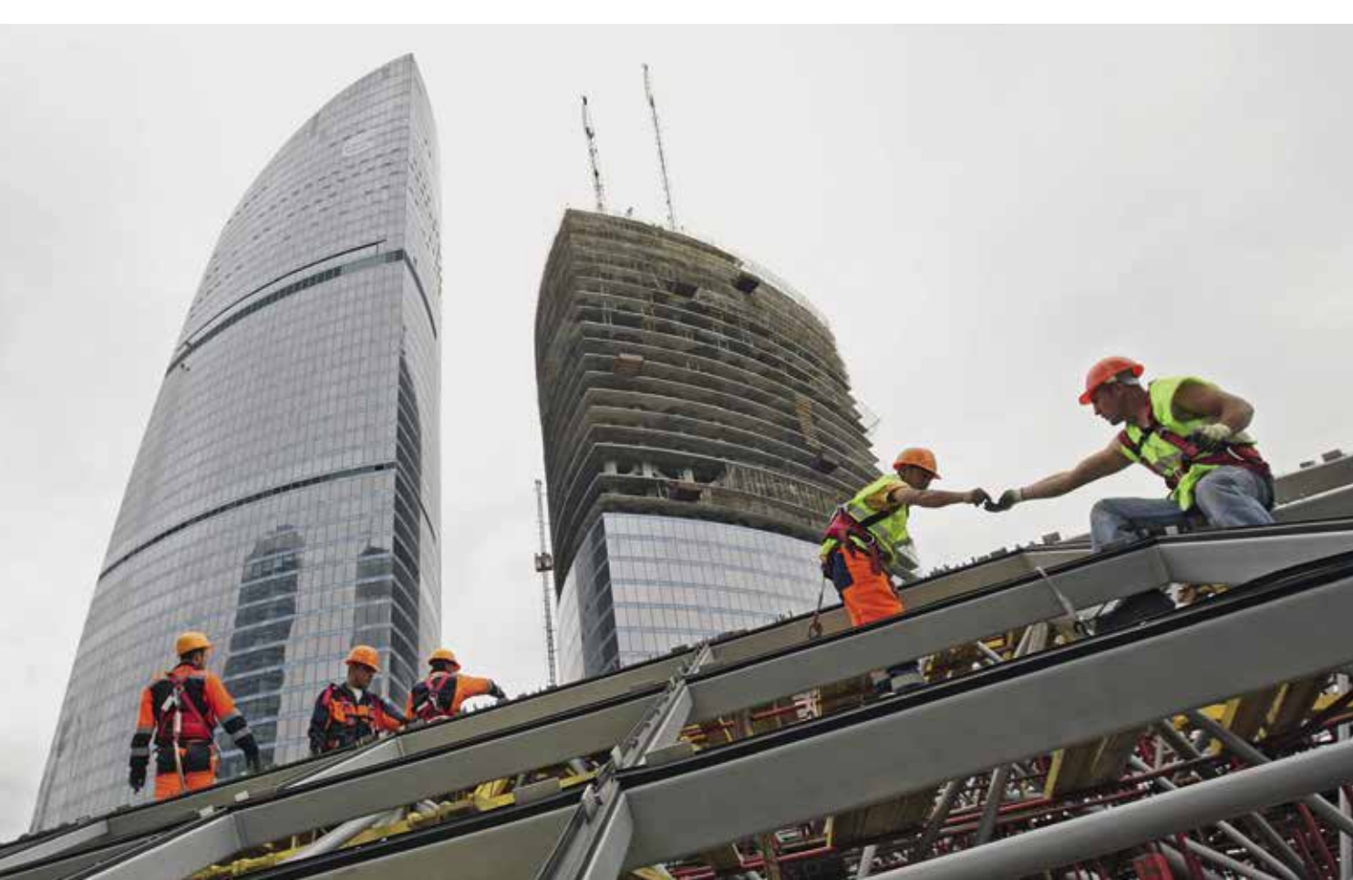
RUSSIA, Moscow. Construction of Moscow City. Iliya PITALEV/RIA Novosti/Sputnik
